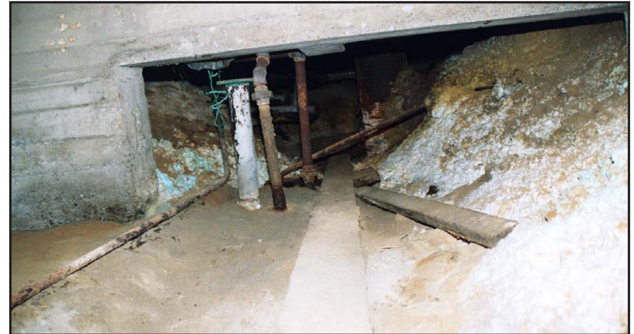
Looking inside crawl space area at location shown to left.
