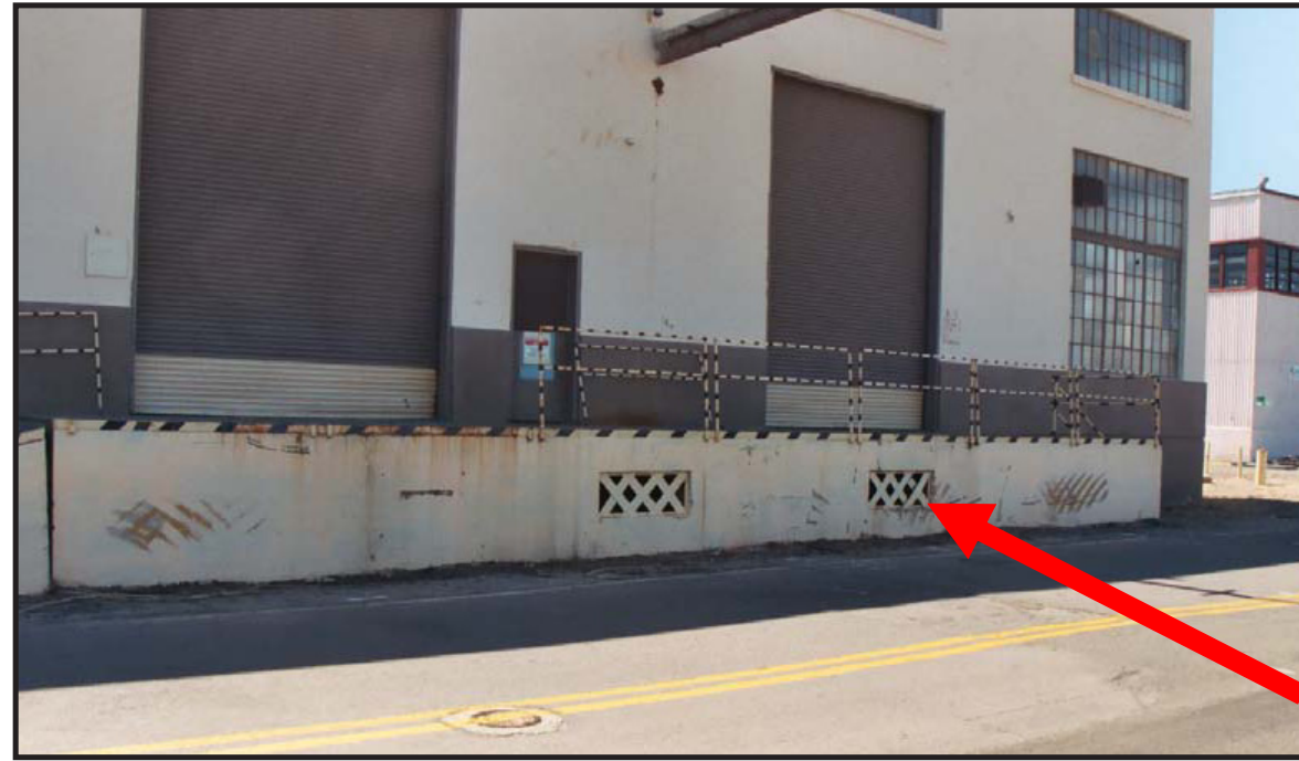
Building 461. Arrow points to location of crawl space.
