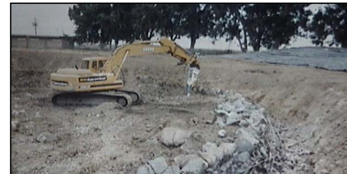
Underground Storage Tank Removal at IR23
