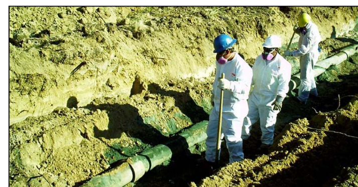
Workers wearing protective gear during ABM and utility removal, Farragut Village
