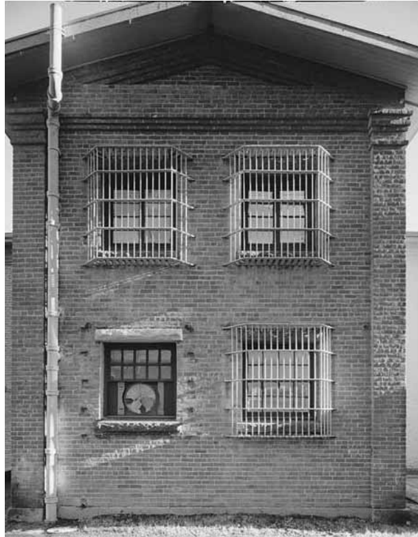
NORTH VIEW OF NORTH WING
