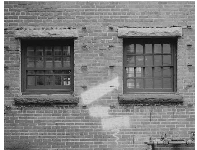
SASH WINDOW W/ CAST STONE SILLS & LINTELS
