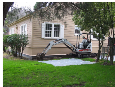
Excavation Work Surrounding Structures East of Azuar Drive
