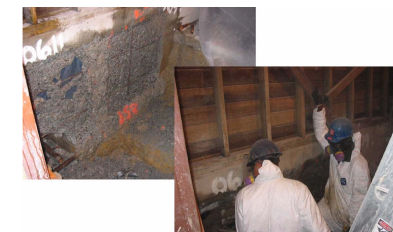
Scabbling in Building H83 to remove PCBs in part of the Concrete Wall on East Side of the building
