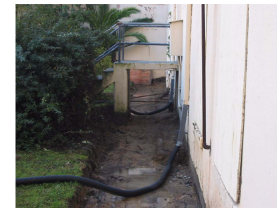
Runoff Controls in place following Excavation around building in Touro University
