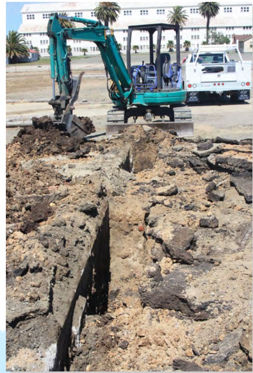
Former Building 531 Vault - ABM Removal Confirmation
