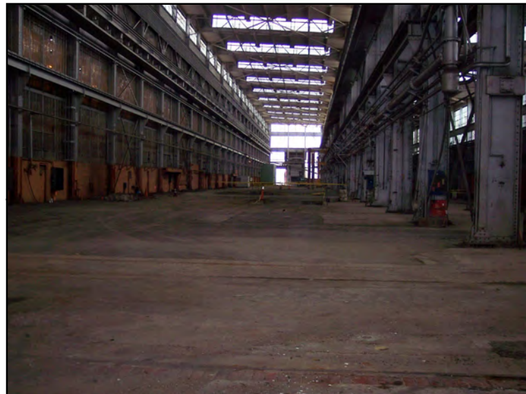
Upcoming Work - Building 386 Oil Pipes Phase I Investigation
