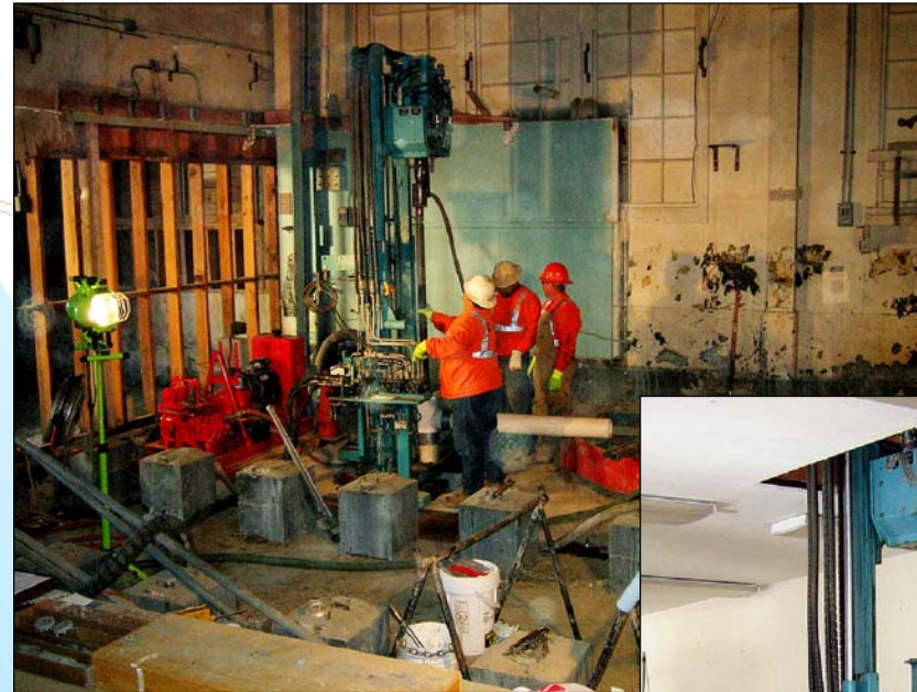
Monitoring Well Installation Inside Building 225
