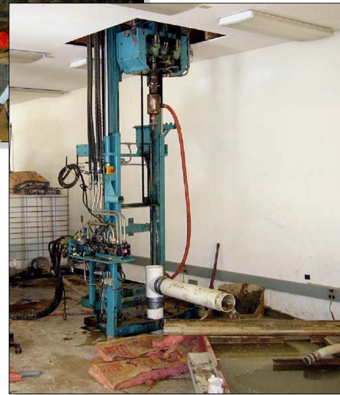
Closeup of Limited Access Sonic Drill Rig
