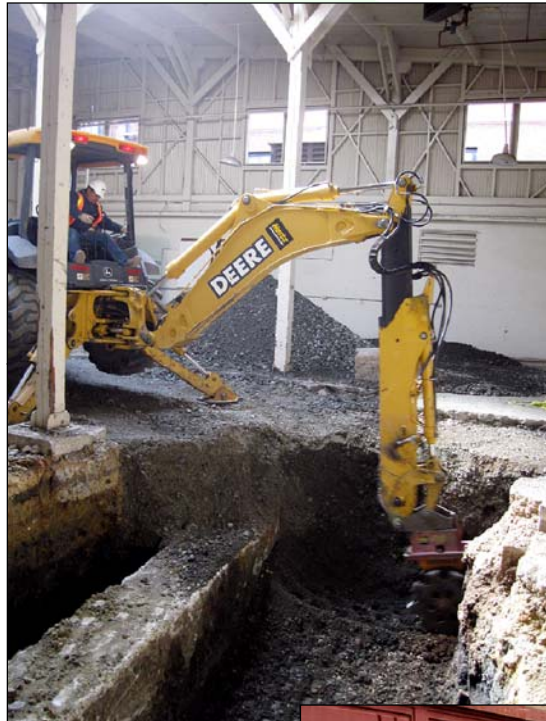
Overexcavation at FOPL H1.6.B85.EX02
