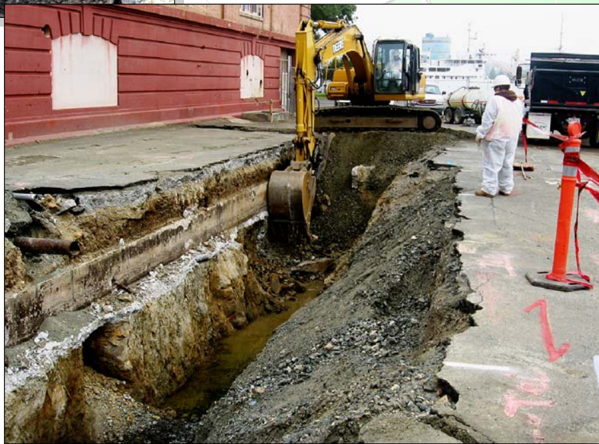
Trenching along FOPL Segment on South Side of B121
