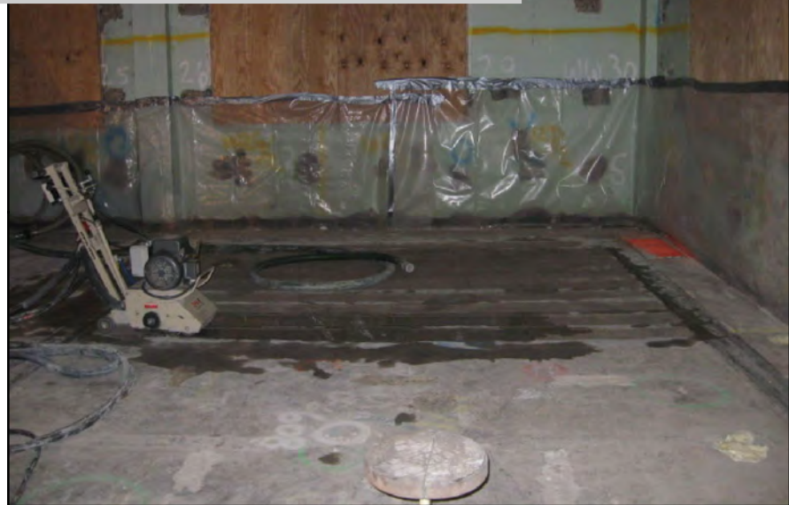
Additional Scabbling Performed at Building 746 PCB SITE AL#03
