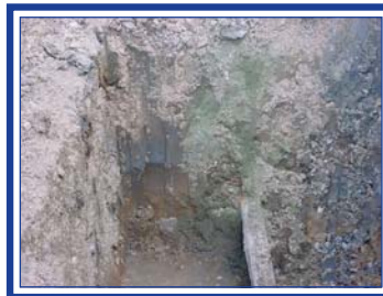
The photographs show the former industrial wastewater pipeline. The green-colored material is sandblast grit referred to as greensand.
