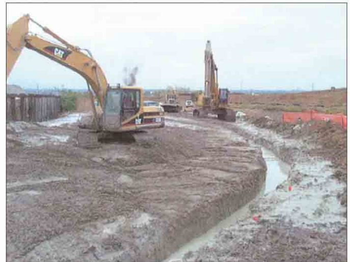
Figure 3. A typical bentonite slurry-filled trench prior to backfill with soil-bentonite mixture.
