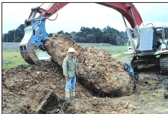
Dredge Pond Outfall Debris Mass
