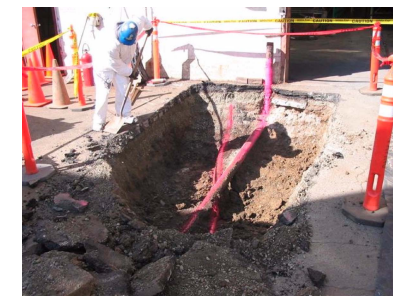
Soil Removal at FOPL Segment on South Side of Building 388
