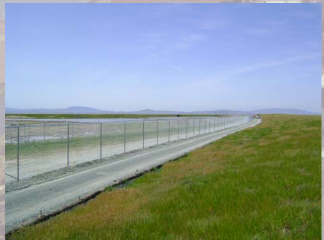
Completed Fence Along Western Perimeter of IA-H1 Containment Area
