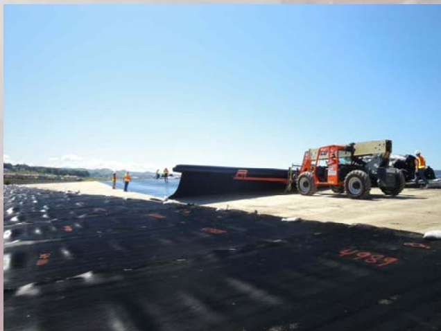
GEOMEMBRANE DEPLOYMENT ACTIVITIES
