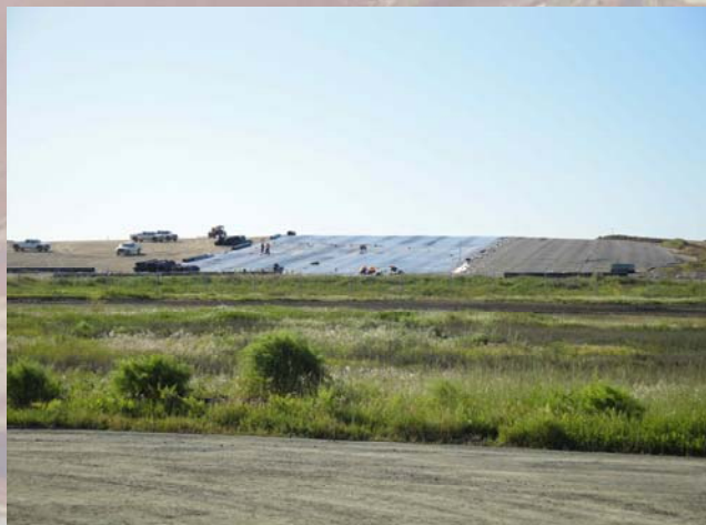
VIEW OF IA-H1 CONTAINMENT CAPPING ACTIVITIES
