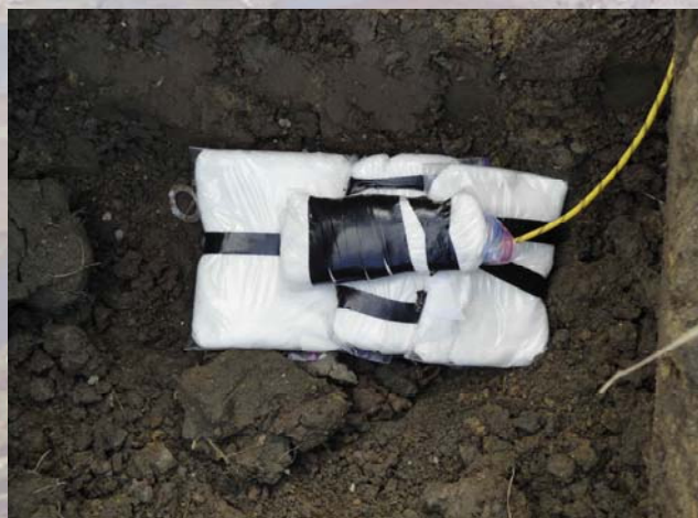
SET-UP SHOT TO DESTROY RECOVERED MEC ITEMS
