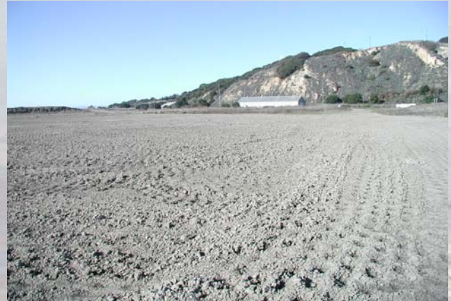
Backfilled portion of IR-05 excavation area
