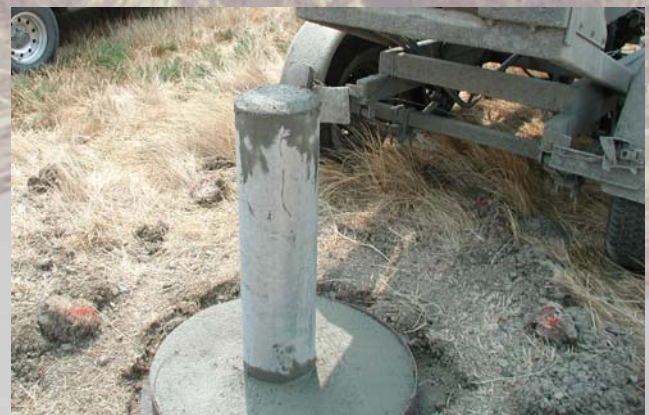
Installation of settlement monuments on the IA-H1 Containment Area engineered cap
