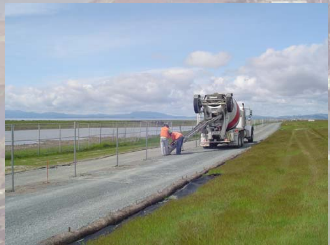
Placement of concrete for fence posts.
