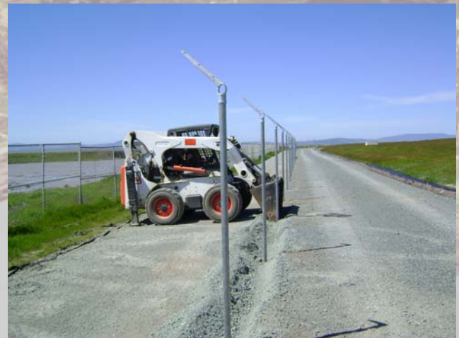
Excavation of 6-inch trench to bury fence fabric.
