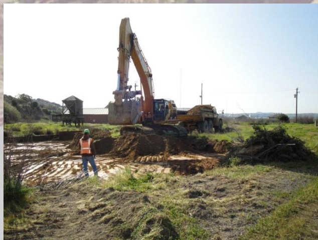
Excavation at the Horse Stable Area within the Western Magazine Area
