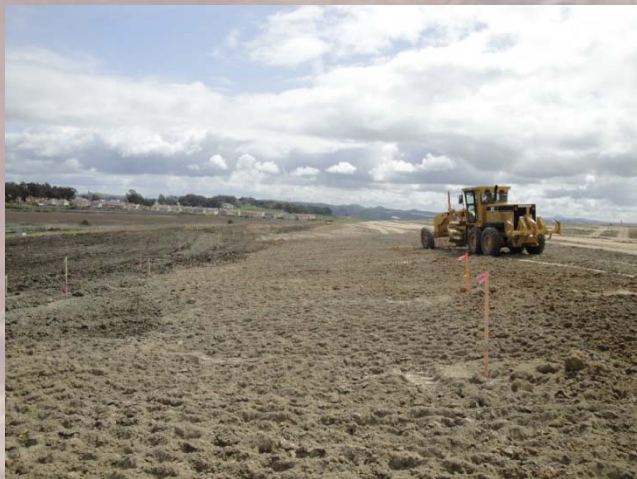
Final Grading Prior to Placement of Geosynthetic Layers
