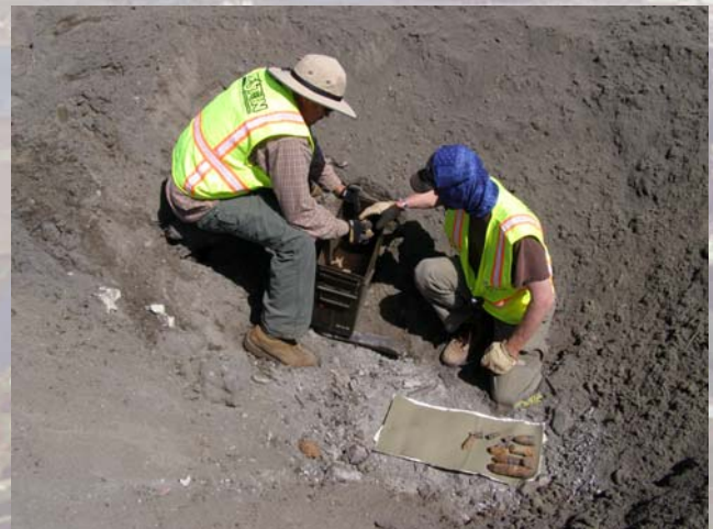
Preparing munitions items for detonation using commercial explosives (flex sheet) before adding several feet of cover sand
