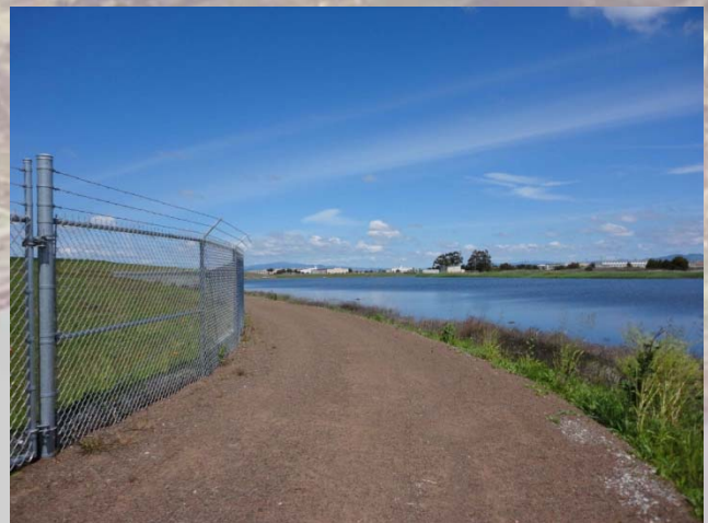
Portion of trail adjacent to eastern wetlands
