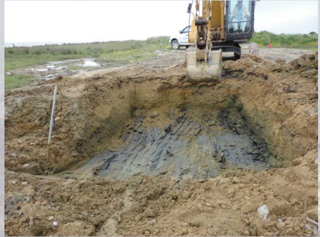
Excavation to remove diesel contaminated soil at IR05
