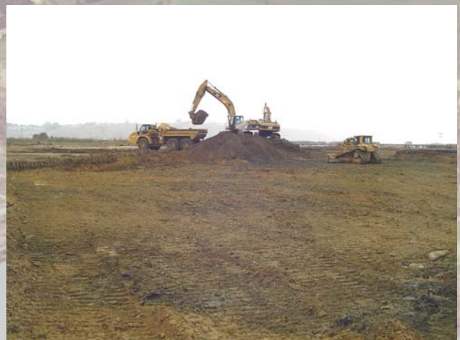
View of excavation activities at IR-05
