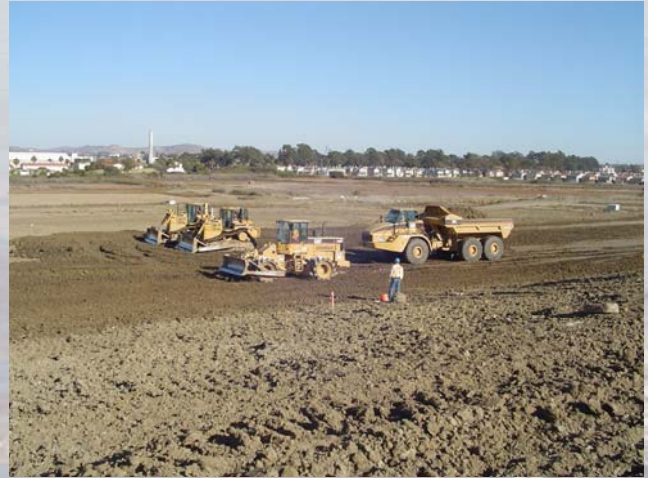
Subgrade grading activities using haul trucks, bull dozers, and soil compactors
