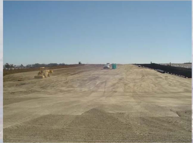
Subgrade preparation prior to installation of geosynthetic layers
