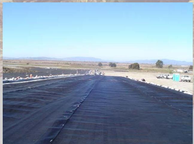
Installation of geosynthetic layers in progress
