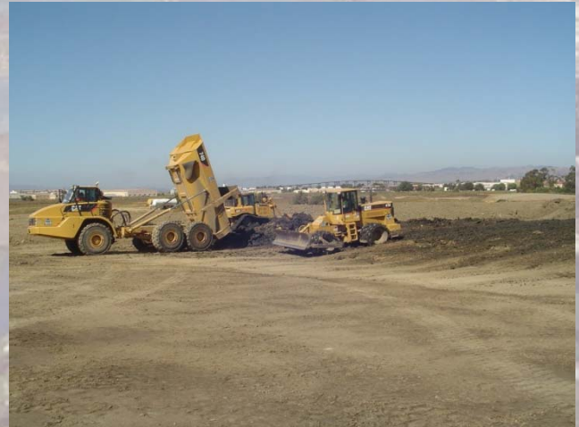
PLACEMENT OF FILL MATERIAL AT IA-H1 CONTAINMENT AREA
