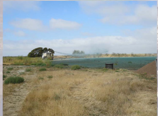
Hydroseeding of the former Fire Fighting Training Area
